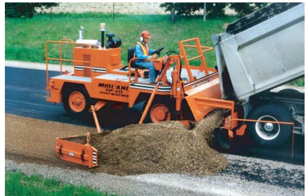
Deep and wide strike off shoulder spreading in one pass
