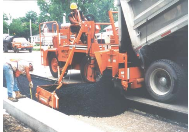
Spread binder layer below grade
