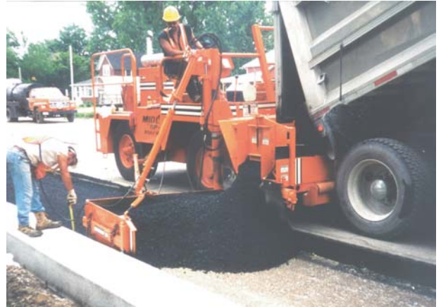
Spread binder layer below grade
